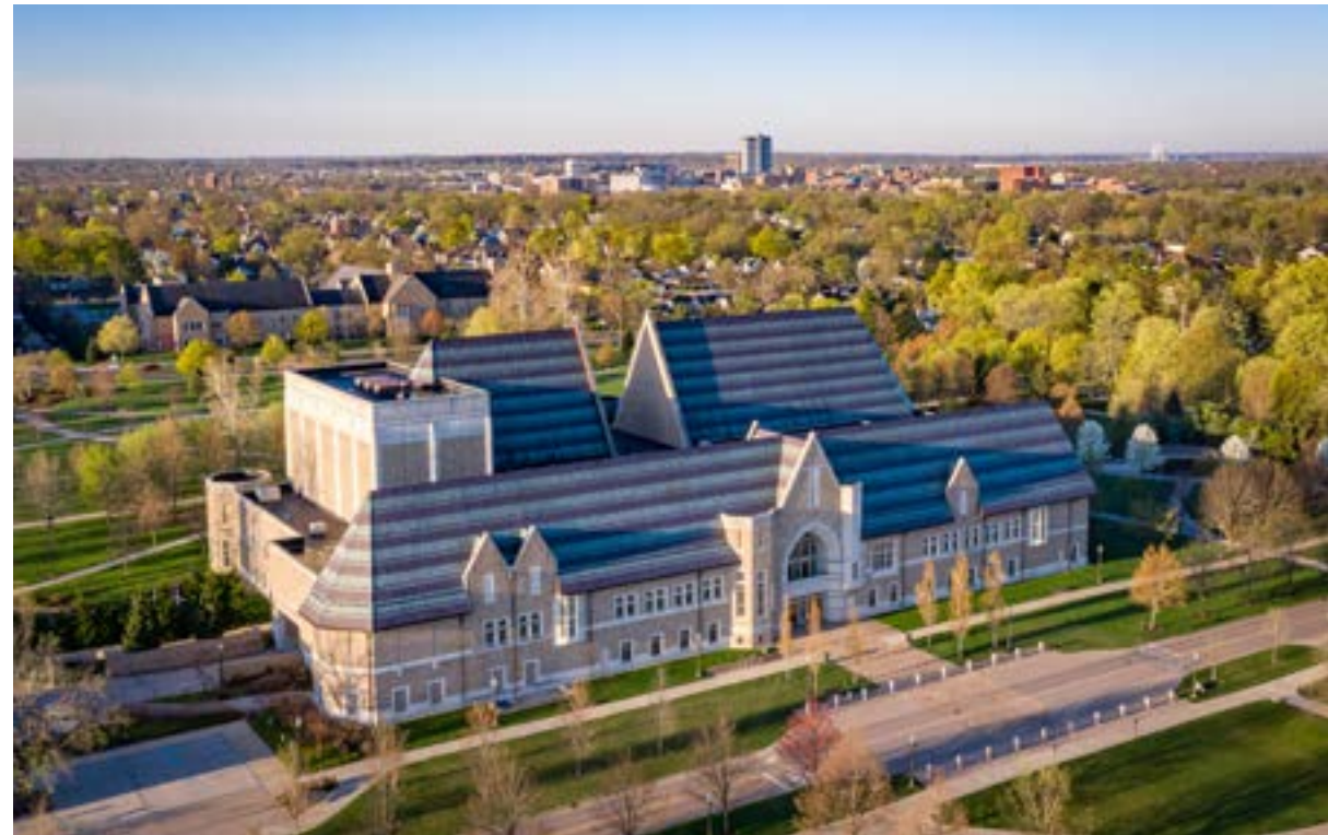
DeBartolo Performing Arts Center, looking south towards South Bend
